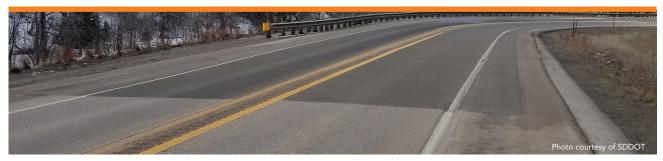
HFST applied at horizontal curve on US Highway 14A through Boulder Canyon west of Sturgis, South Dakota.
