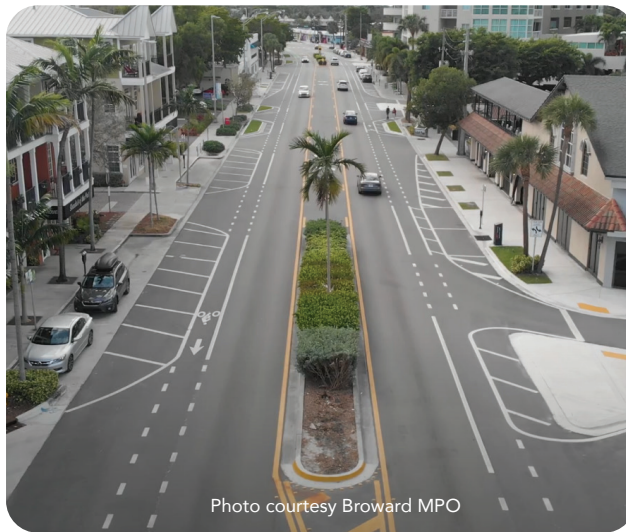
Aerial view of Wilton Drive showing on-street parking, buffered bike lanes, median separation, and pedestrian facilities.
