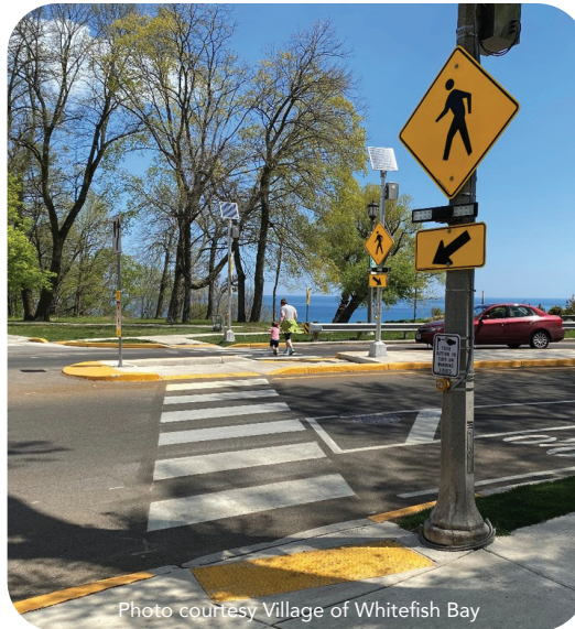
Photo courtesy Village of Whitefish Bay “Danish Offset” crossing at a curve on Lake Drive at Palisades Road.
