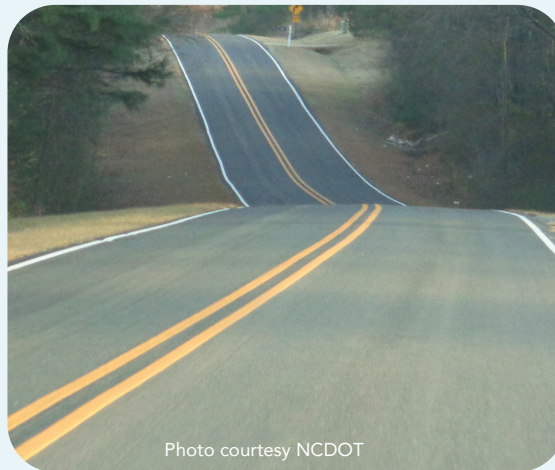
An application of long-life double centerline markings on North Carolina State Route 1131.
