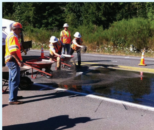
Installation of high-friction surface treatment (HFST) – example improvement resulting from the county safety program
