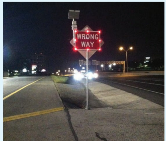
LED illuminated Wrong Way sign with radar – standard wrong-way driver countermeasure on exit ramps in San Antonio for deterring wrong way drivers
