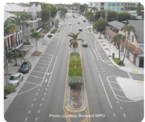
View of Wilton Drive showing on-street parking, buffered bike lanes, median separation, and pedestrian facilities.
